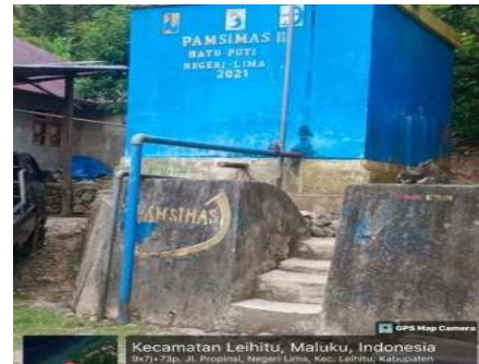
Gambar 7. Bak Reservoir
